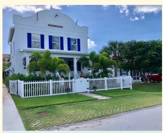
Turf block, shown in the right-of-way area immediately bordering the street in the photo above, has been used in certain developments in the Bayshore neighborhood to allow for use of right-of-way space for parking. This option should be evaluated as part of the right-of-way design considerations in the stormwater master plan update.
