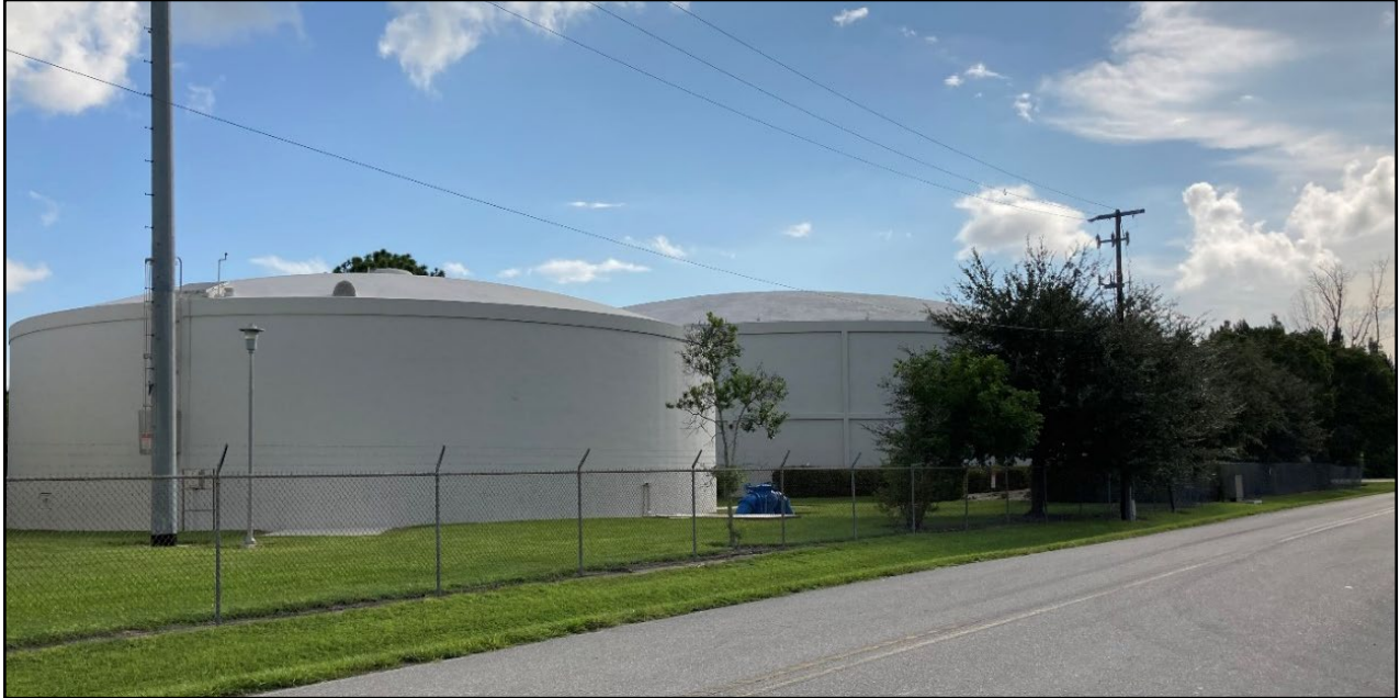
Water Towers – Gateway Triangle Area
