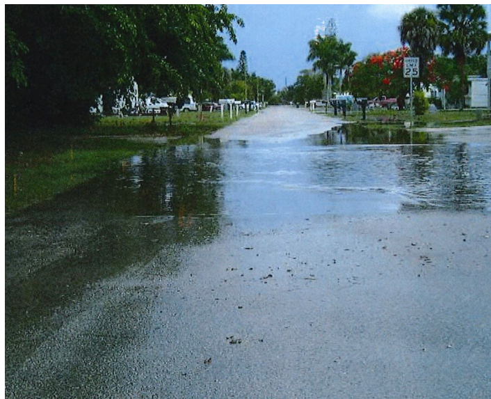
Stormwater improvements are ongoing to alleviate street flooding
