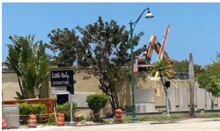
Iconic Little Italy Demolition
