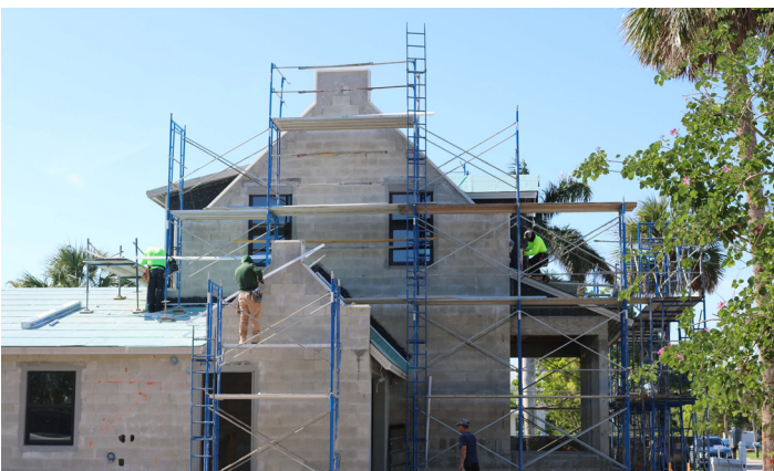
Residential house under construction on Jeepers Drive
