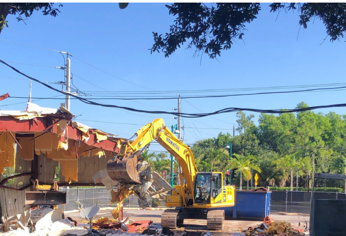
Demolition process of the buildings
