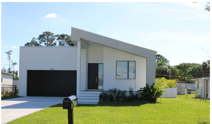
New house completed on Karen Drive, 1 of 6 houses built on the scattered lots
