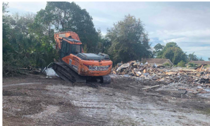
Demolition of existing structure on Francis Avenue lot
