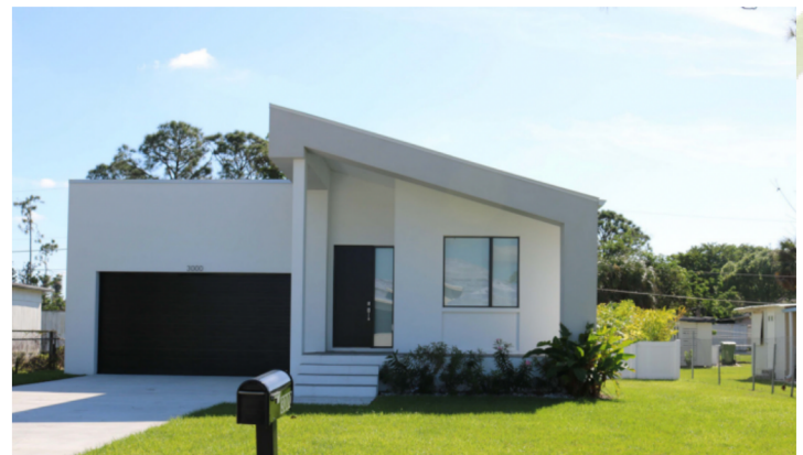
New house completed on Karen Drive, 1 of 6 houses built on the scattered lots
