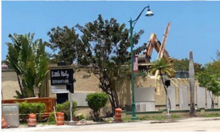
Iconic Little Italy Demolition
