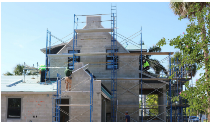
Residential house under construction on Jeepers Drive
