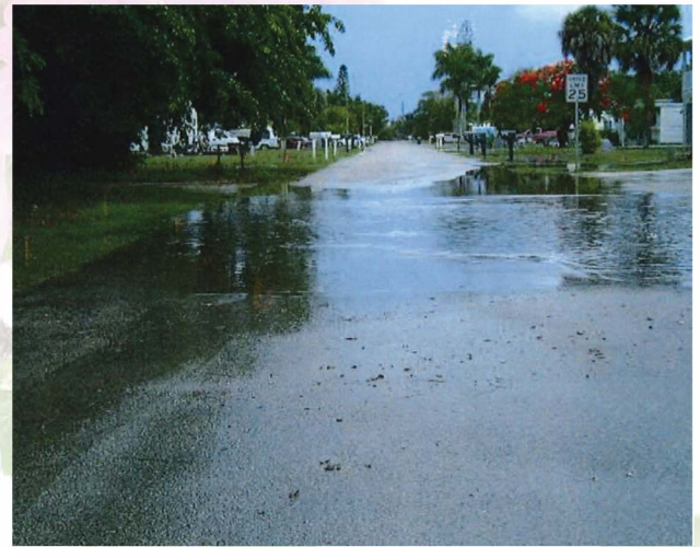
Stormwater improvements are ongoing to alleviate street flooding
